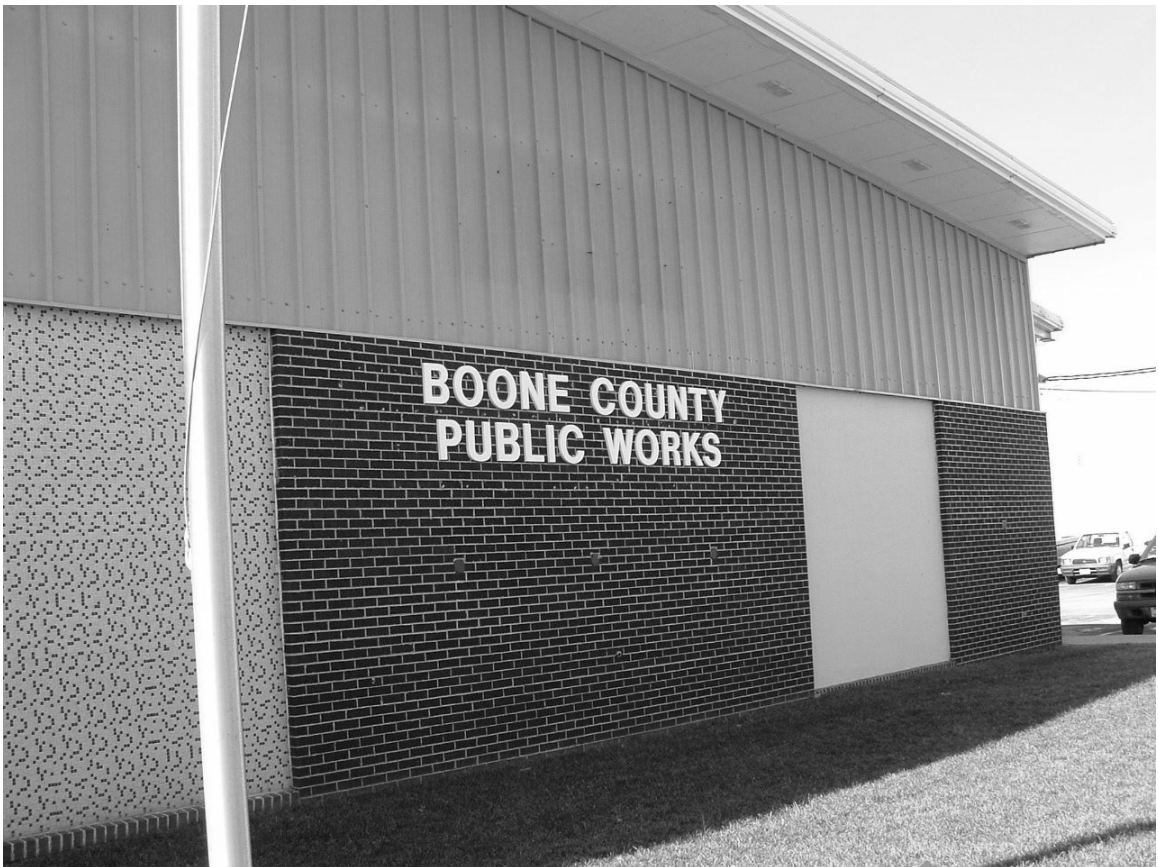
MAINTENANCE BUILDING – EAST ELEVATION
