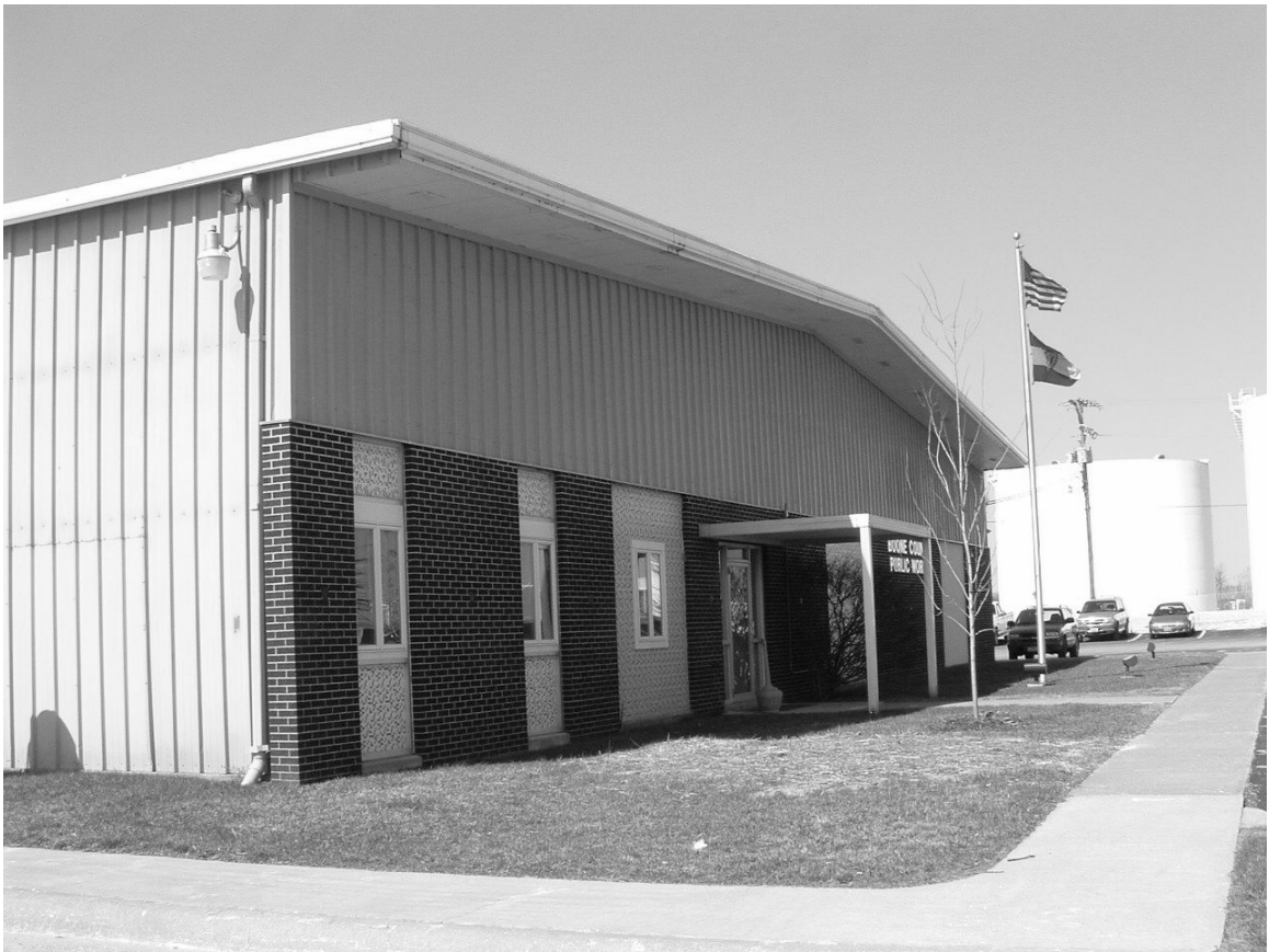
MAINTENANCE BUILDING – EAST ELEVATION
