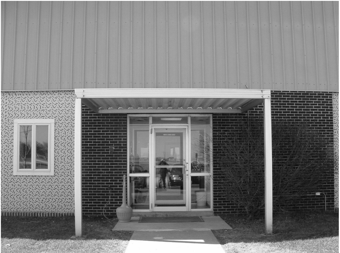
MAINTENANCE BUILDING – CANOPY AT EAST ENTRANCE
