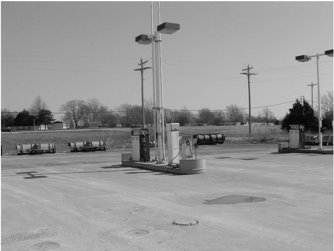
CENTER AND SOUTH FUEL ISLANDS
