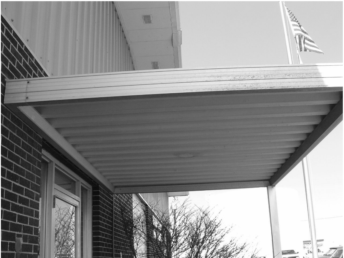
MAINTENANCE BUILDING – CANOPY AT EAST ENTRANCE
