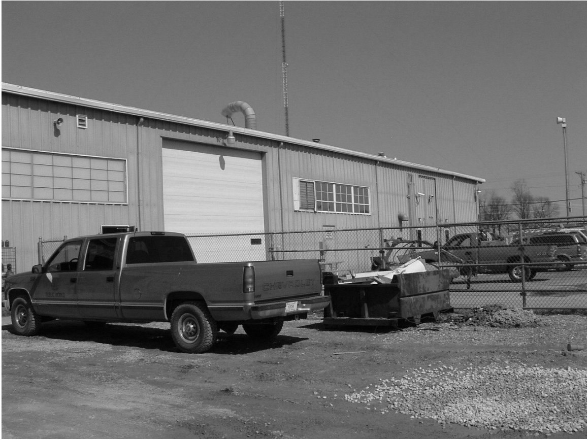
MAINTENANCE BUILDING – SOUTH ELEVATION
