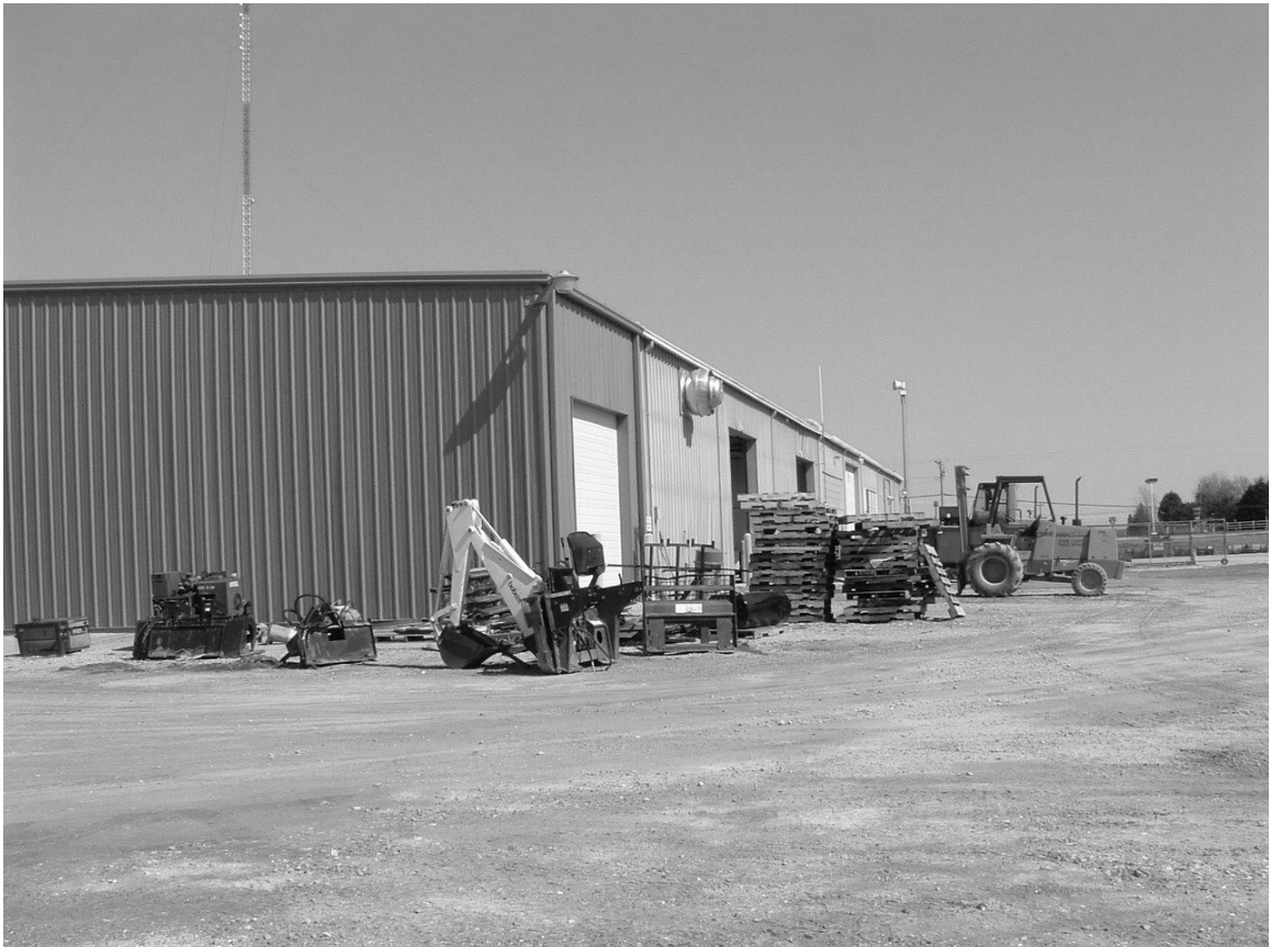
MAINTENANCE BUILDING – SOUTHEAST CORNER
