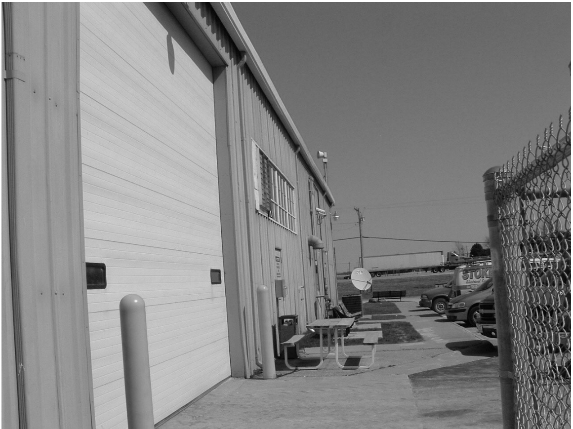
MAINTENANCE BUILDING – SOUTH ELEVATION
