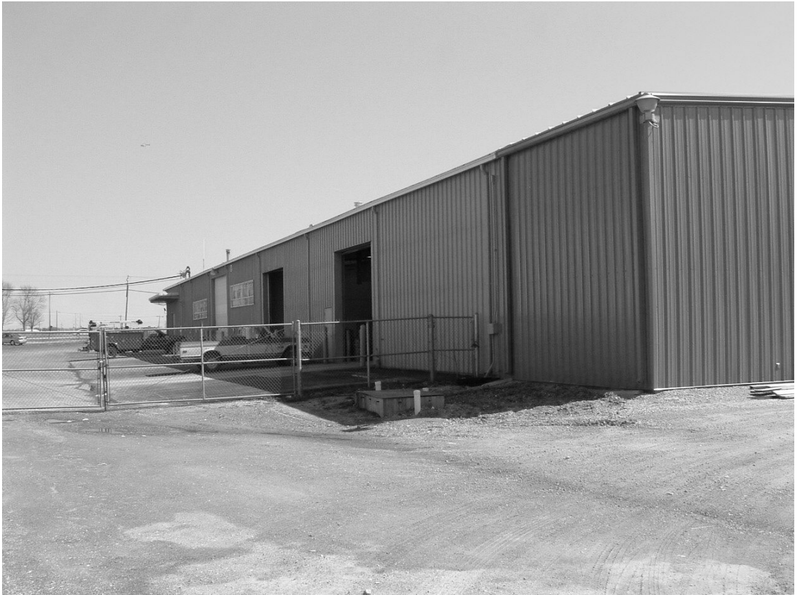
MAINTENANCE BUILDING – NORTHEAST CORNER
