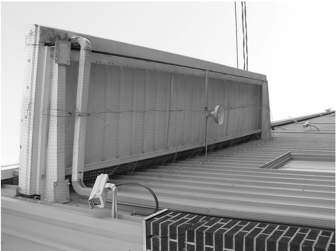
MAINTENANCE BUILDING – NORTHEAST CORNER
