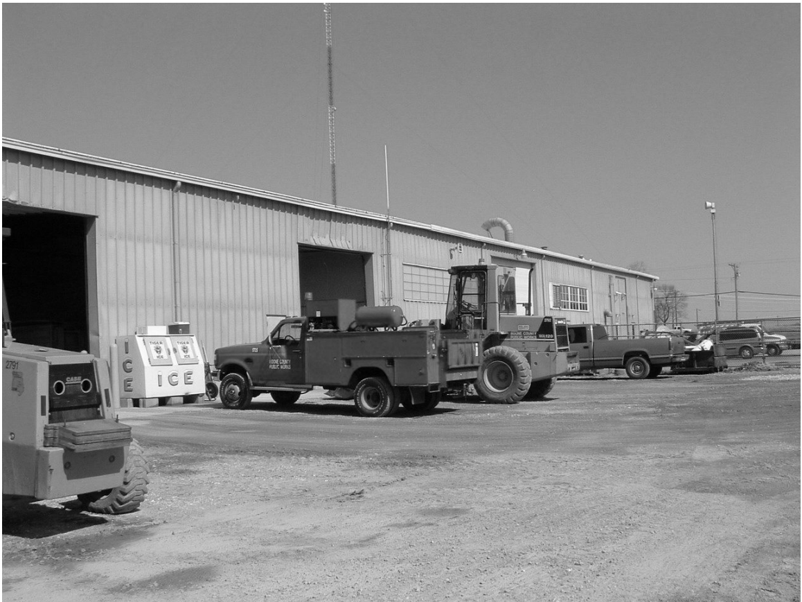
MAINTENANCE BUILDING – SOUTH ELEVATION
